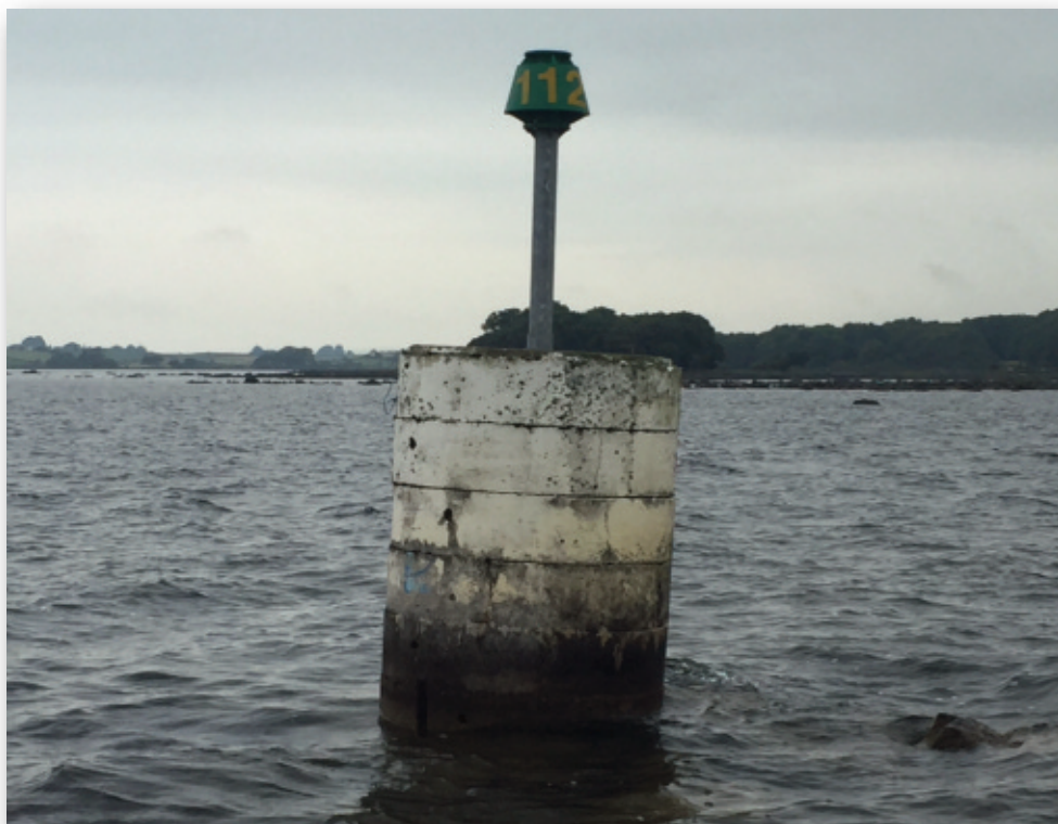
Photograph No. 1: Lough Corrib Navigation Marker No.112.
